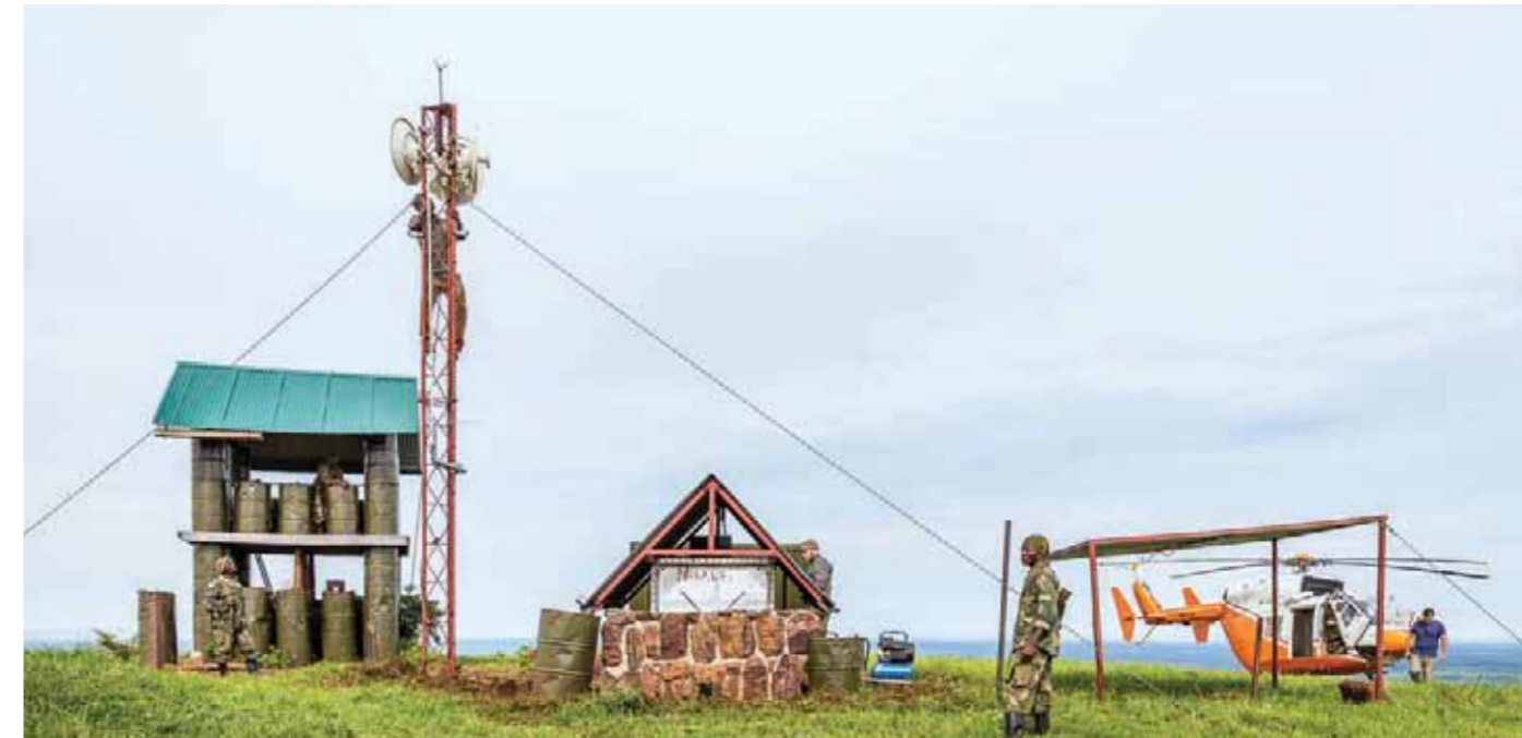
Infrastructure is a critical foundation to support all park functions. © Marcus Westberg
